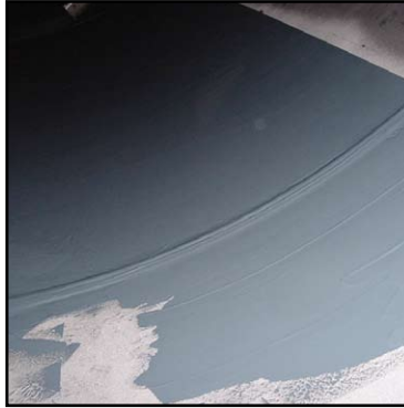
The Belzona® 1391 being applied.
