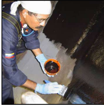
View of the application underway. Belzona ® 1121 and Belzona ® 5891 were used.
