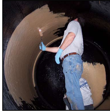
Contractor applying 2nd coat of Belzona® 5811
