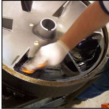
New prepared slinger being wetted out with Belzona® 2131
