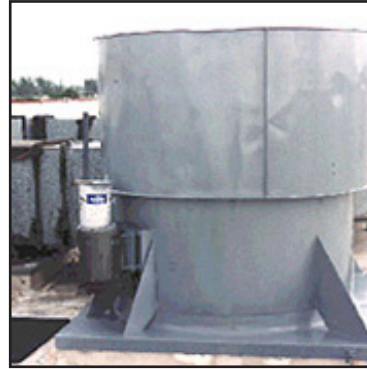
Completed coating with Belzona® 5111 (Ceramic Cladding)
