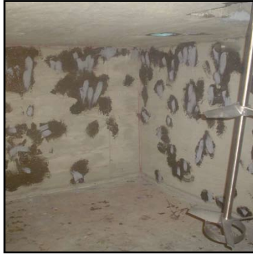
Surface prepared and holes patched with Belzona® 4111
