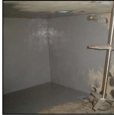
First coat of Belzona® 5811 being applied
