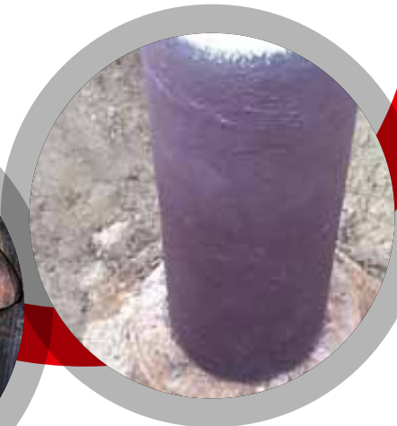
Repair of Thin Wall Defects
