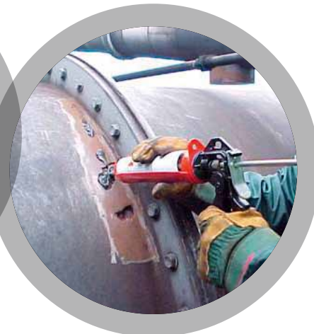
Filling of Corrosion Pits
