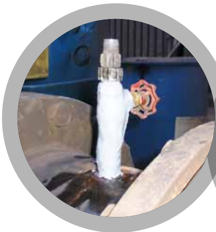
Leak Sealing of Pipework
